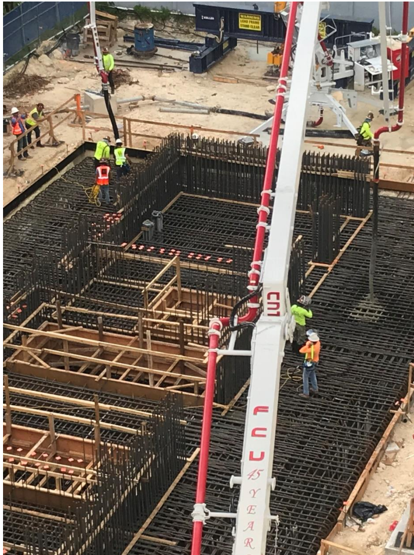
YOTELPAD MIAMI, BEFORE THE POUR, IMAGE VIA ARIA DEVELOPMENT GROUP
