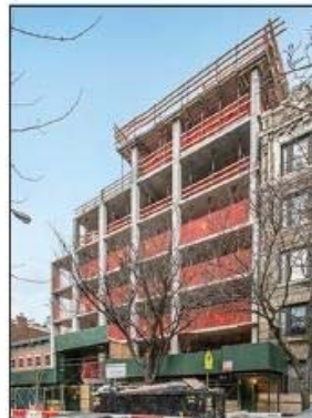
Superstructure of 465 Pacific Street tops out.
